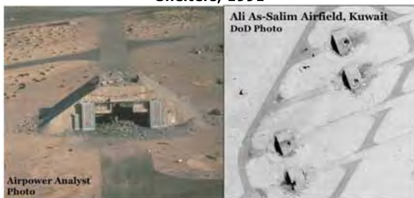
Figure 24: LGB Damage against Hardened Aircraft Shelters, 1991
