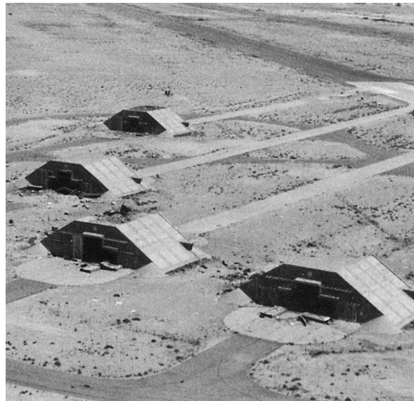
Figure 4: Hardened Aircraft Shelters in Al Jaber Airfield, Kuwait
